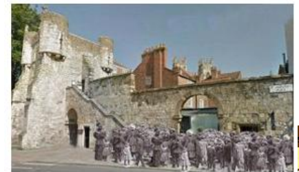
Restoration of York City Walls
