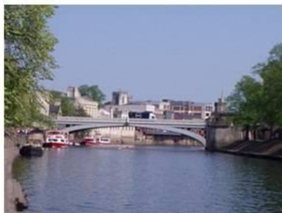
Lendal Bridge, York
