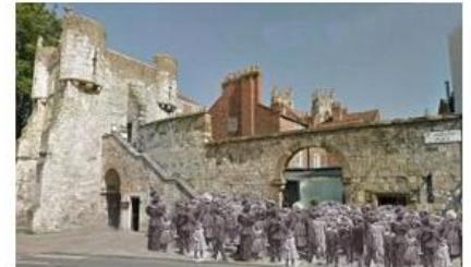
Restoration of York City Walls
