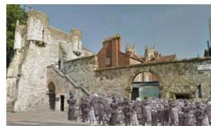
Restoration of York City Walls
