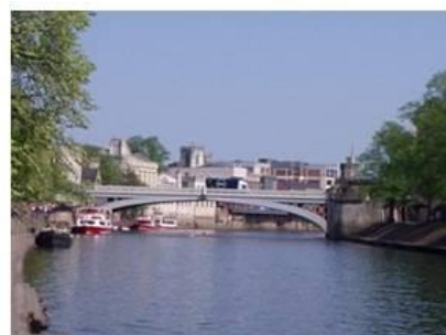
Lendal Bridge, York
