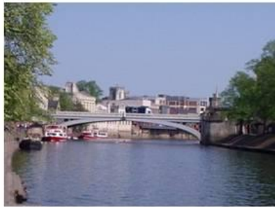
Lendal Bridge, York
