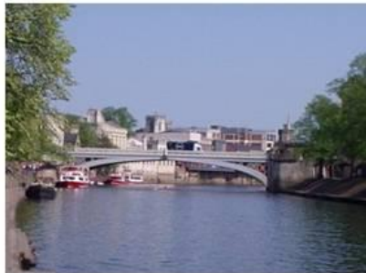
Lendal Bridge, York
