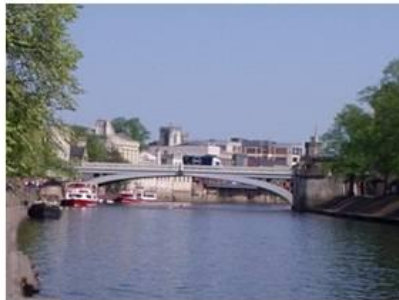
Lendal Bridge, York
