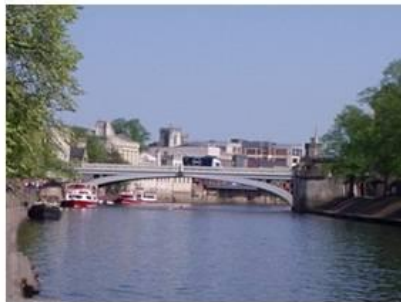
Lendal Bridge, York
