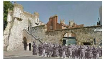
Restoration of York City Walls
