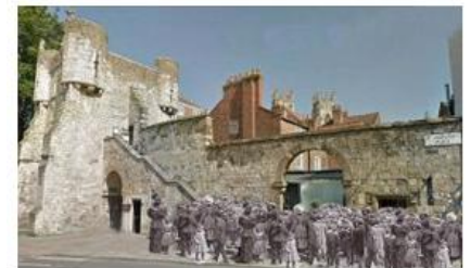
Restoration of York City Walls
