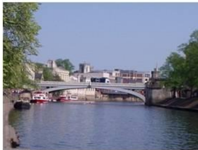
Lendal Bridge, York
