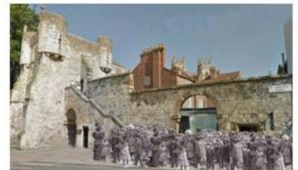
Restoration of York City Walls
