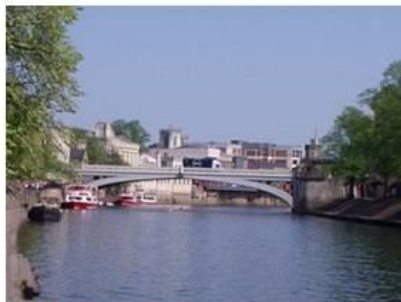
Lendal Bridge, York
