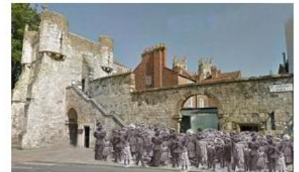
Restoration of York City Walls
