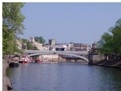
Lendal Bridge, York
