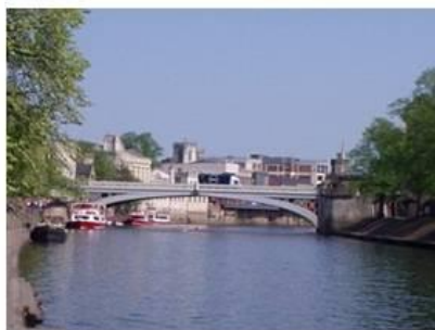
Lendal Bridge, York
