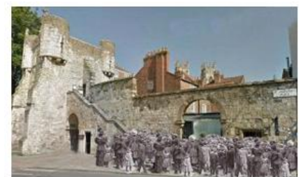
Restoration of York City Walls
